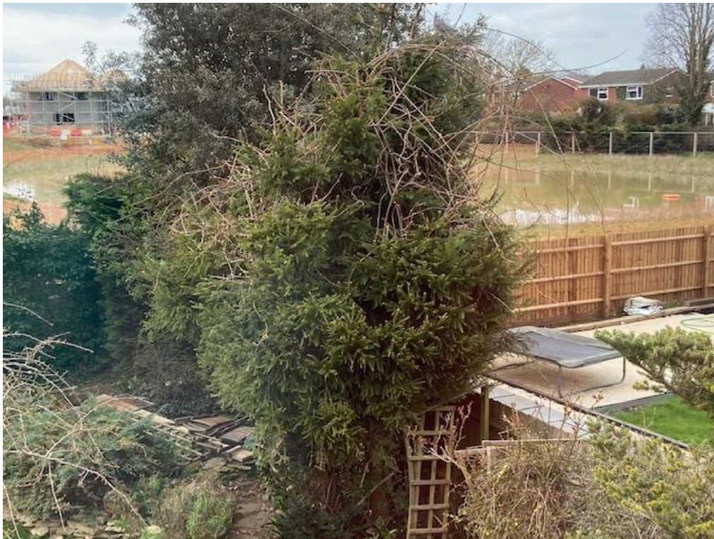
Figure 2-Photo of the attenuation basin taken by the resident on 20th March. It shows one of the attenuation basins on the Bloor development that has now been flooded, as stated by the resident, for 7 consecutive months.
