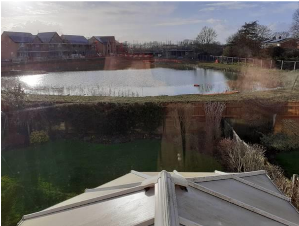
Figure 1- Photo showing Attenuation Basin solution filled by groundwater infiltration on the similar Buckden Lucks Lane site. Note that the level of water is higher than the surrounding houses/gardens.
